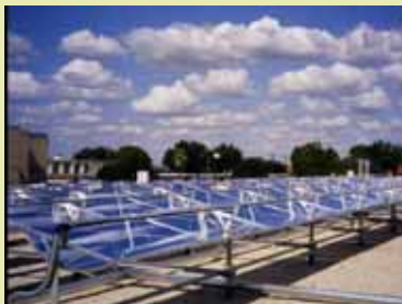
Source: Industrial Solar Tech
